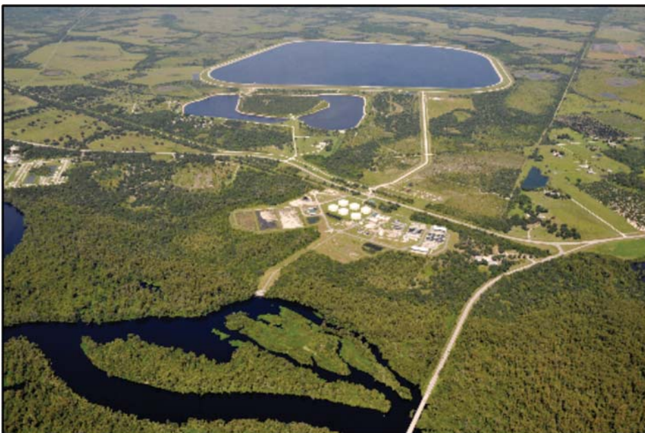
Figure 1. The Peace River Facility With Reservoirs Looking West Over the Peace River
